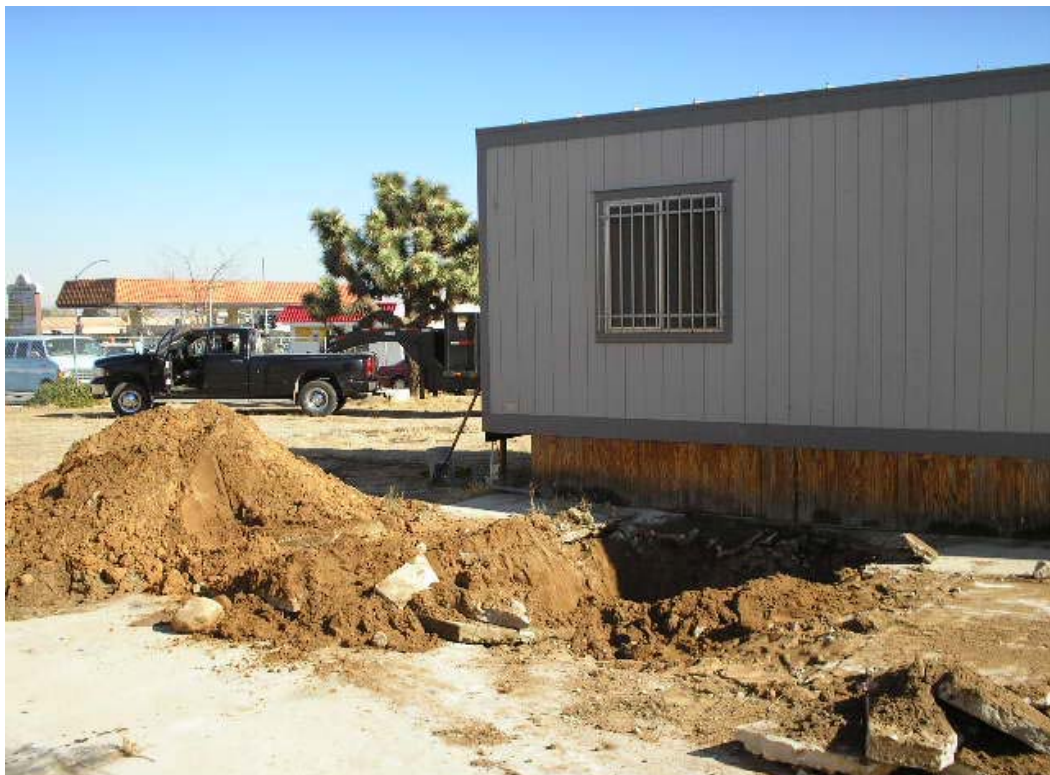
Photograph Number 8: Hydraulic lift removal excavation behind portable building in SW corner.
