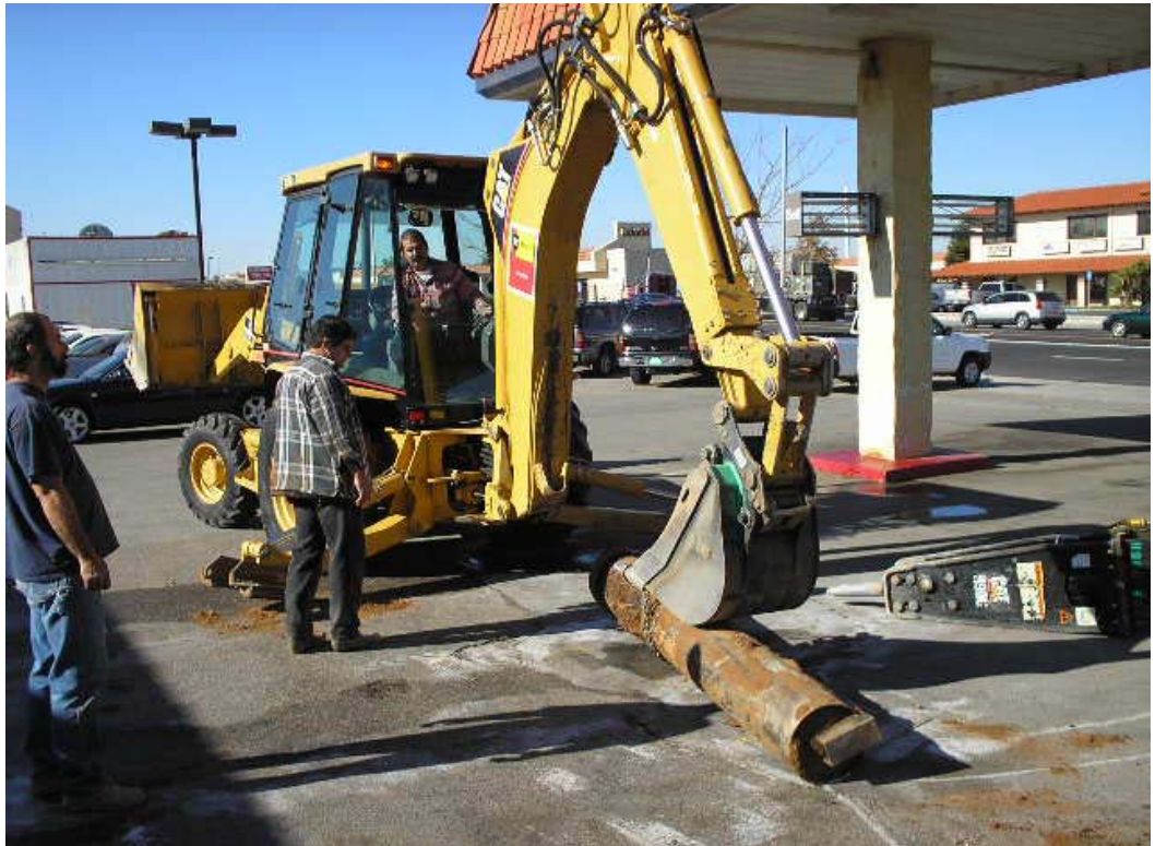
Photograph Number 5: Hydraulic lift cylinder removed from garage
