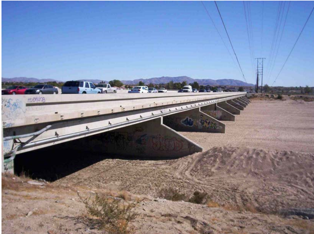
Figure 3-4: Bear Valley Road Bridge Across the Mojave River
