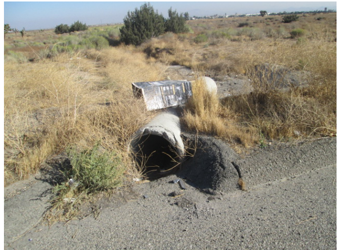
View of representative drain conduit on southern property line
